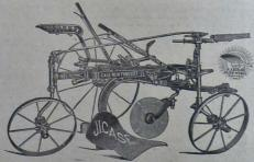
THE J. I. Case New Foot Lift Sulky and Two and Three-bottom games are companion plows, the principle of construction and adjustment of each being identical The games are built heavier in proportion to stand he strain to which they are subjected.
