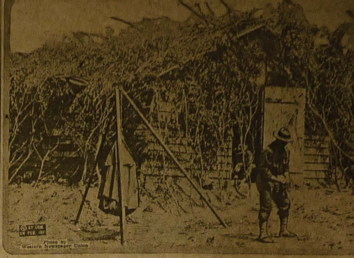
The hits of the American marines now training behind the lines in France have been covered with brushwood to keep them from being seen by enemy flyers.
