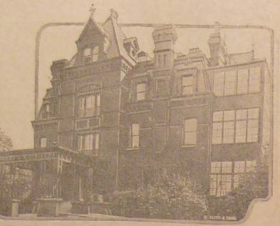
The Japanese embassy has leased this building at Twentieth street and Massachusetts avenue, Washington, for the duration of the conference on the limitation of armaments.
