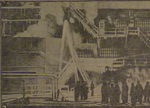
View of the fire at the Atlantic Refining company's plant in Pittsburgh in the course of which seven firemen fell into a huge tank of oil and were drowned.
