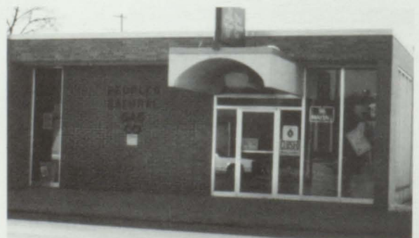
PEOPLE'S NATURAL GAS COMPANY Pine City, Minnesota
