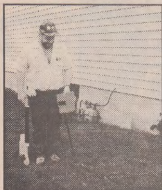
Locating a line is Dennis Vacinek.
