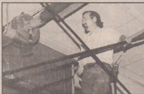
Here Bill Anderson is repairing a commercial heating system.
