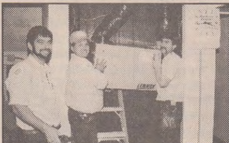
The Installation Crew Hard at Work Left to right: Jay Jahnz, Larry Latourelle and Dale Kirchberg.
