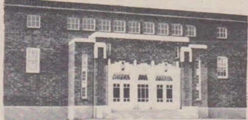
PINE CITY H.S. AUDITORIUM ENTRANCE
