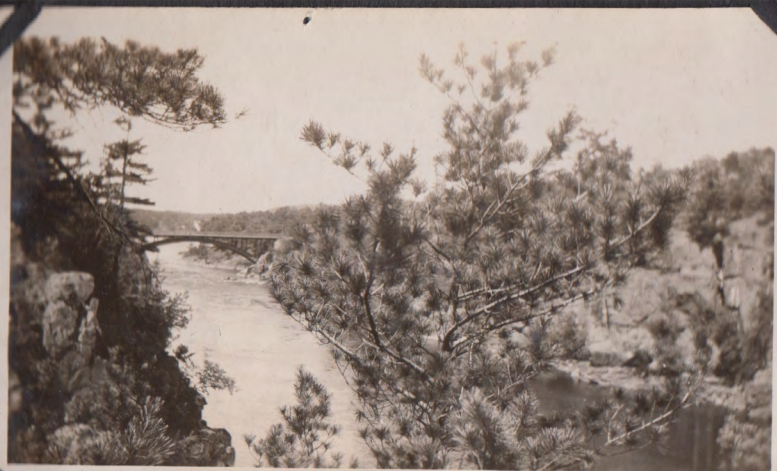
ST. CROIX BRIDGE
