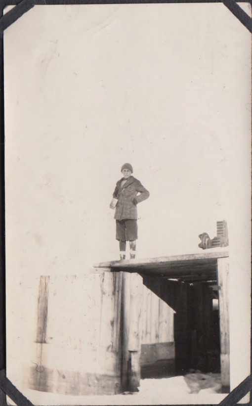
Stub on Fishway
