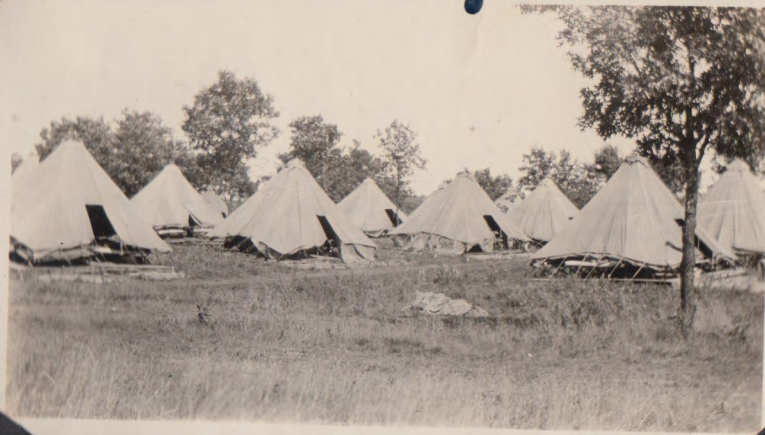
Battery A, B, C.
