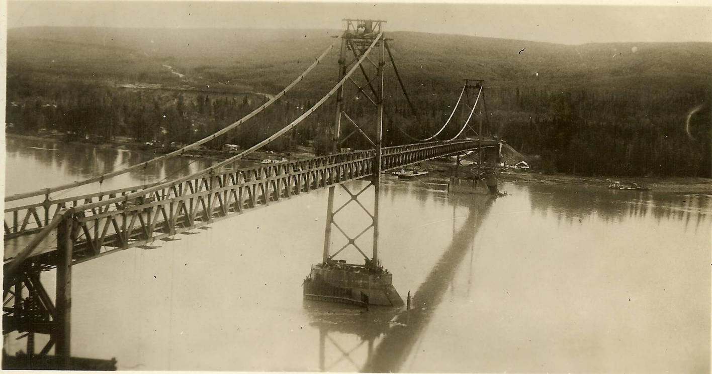
THE ALASKA HIGHWAY Peace River Bridge, between Dawson Creek and Fort St. John Overall length 2,200 feet. cost $1,700,000. Permission of Public Roads Administration ©
