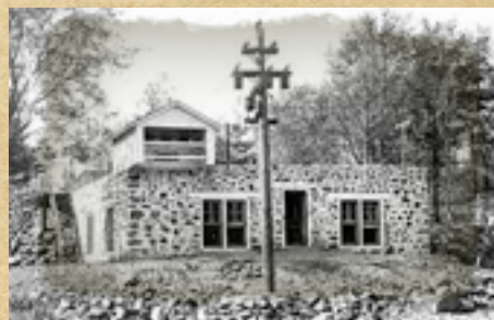
Power Dam House
