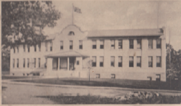
MAIN BUILDING, BLISS ELECTRICAL SCHOOL, YACOWA PARK WASHINGTON, D. C.
