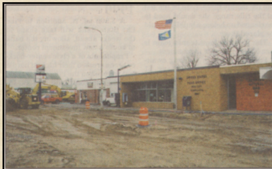
Reconstruction of Highway 61 in the early 2000s.
