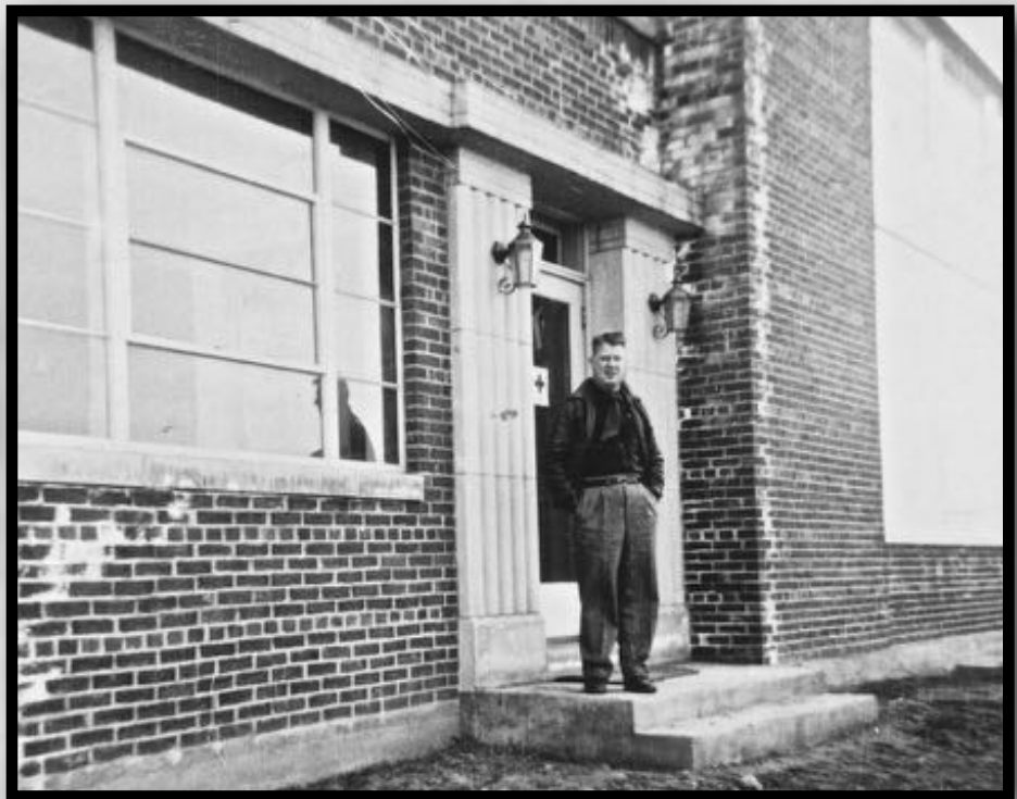
Ed Nelson at new Ashland plant in 1954.
