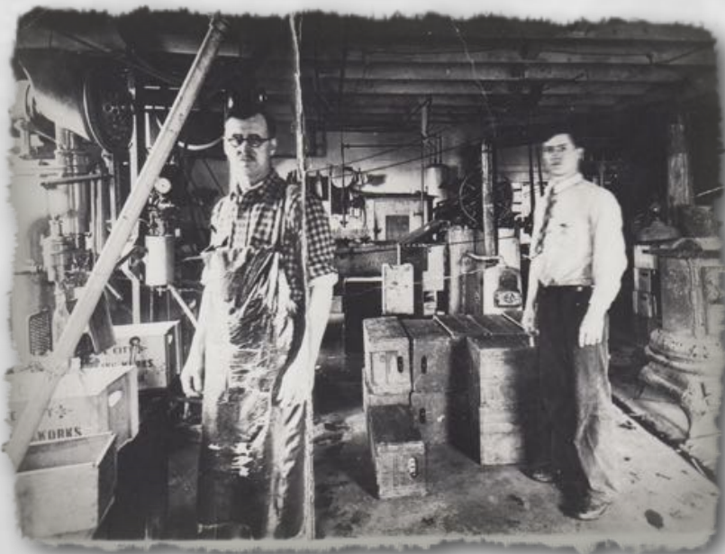
Albert and Art Nelson in the basement of the original Pine City Bottling Works plant.
