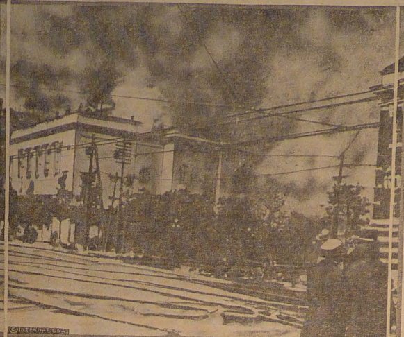
This photograph, taken the day after the first earthquake shocks, shows the conflagration sweeping through Tokyo. In the center is the Imperial theater.
