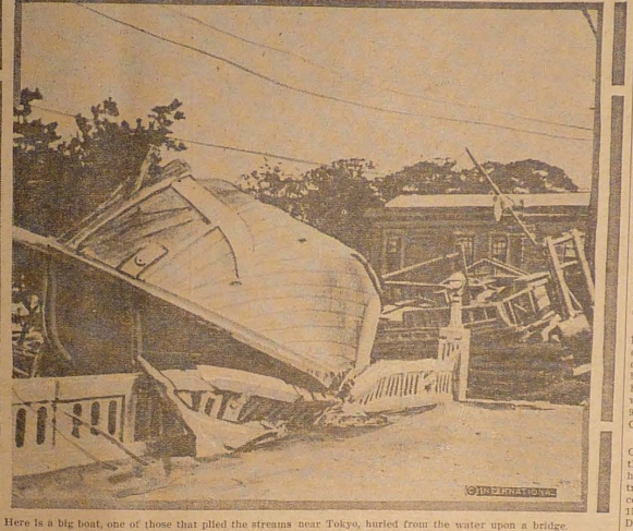
Here is a big boat, one of those that piled the streams near Tokyo, buried under the water upon a bridge.
