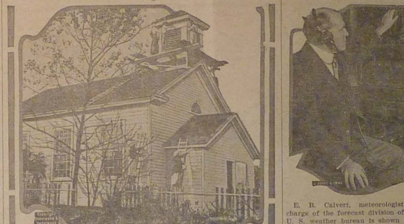
When recently it became necessary to have the Unalaska chapel at East Housatonic, Long Island, repainted the painters wanted too much for the job. So members of the ladies' aid society decided to do the work themselves. Seventeen of them put on overalls and speedily painted the chapel.
