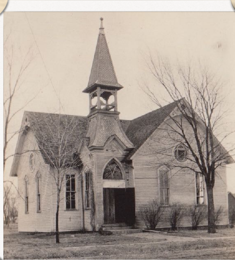
The old church, right before demolition.
